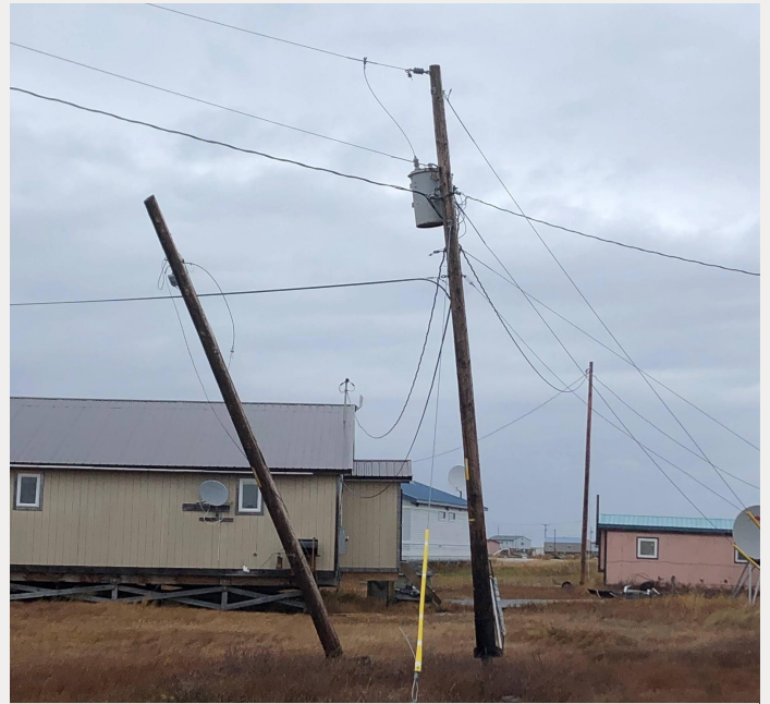
Power lines leaning precariously. Failure of these lines and poles could cause serious harm to people and homes.
