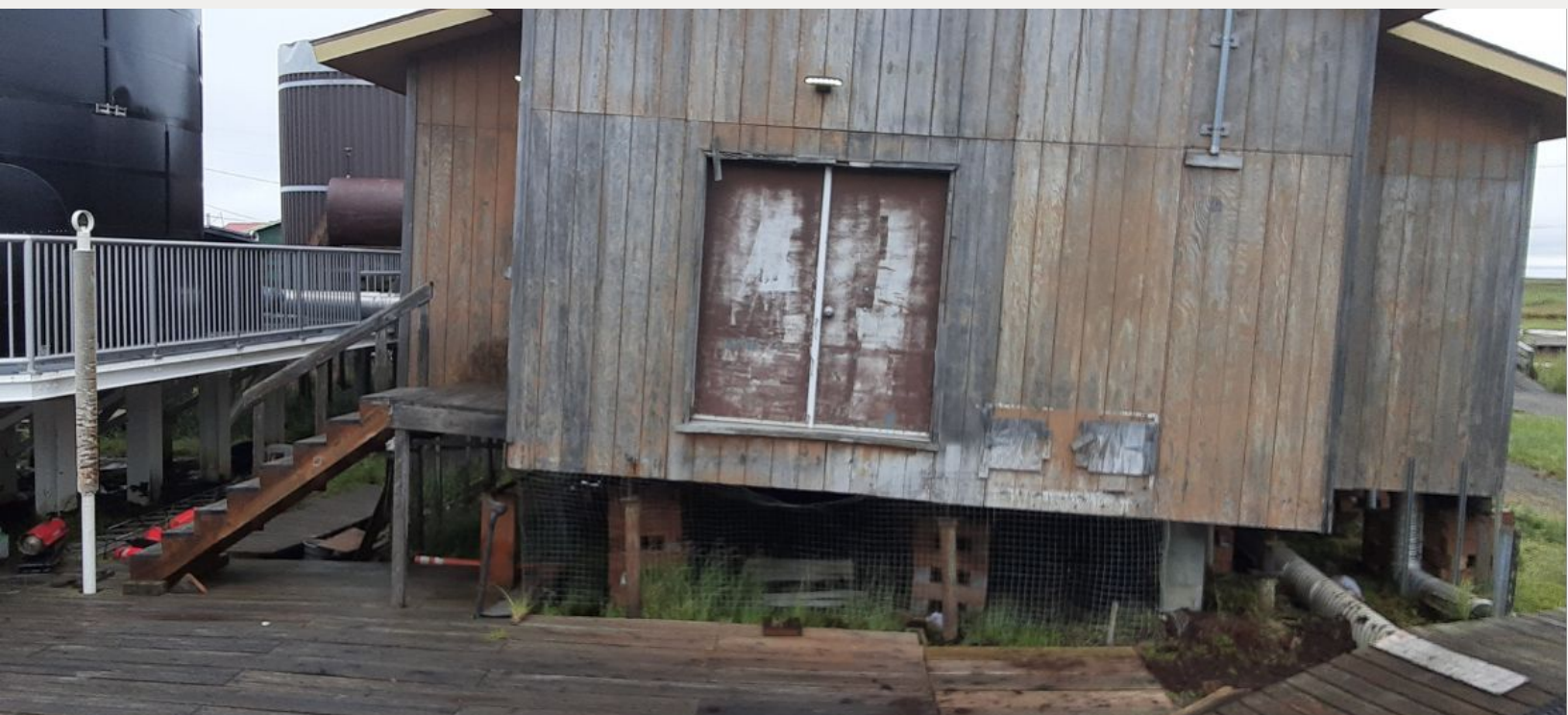
Obvious signs of ground and foundation failure.
