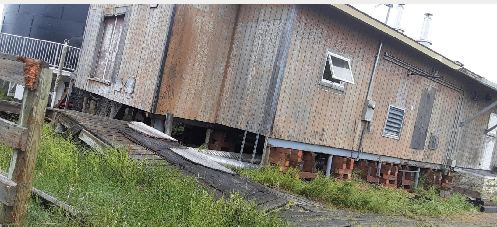
The backside of the building shows mitigation attempts to lift or stall the sinking of the facility. Unfortunately, there is no longer stable permafrost to support its foundation.
