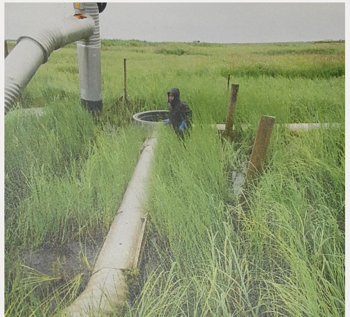
The fresh water system that was built on tundra is now floating on unstable marshy wetland.
