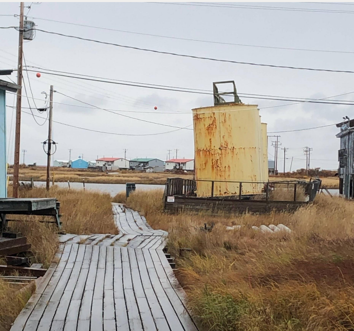
A leaning tank farm is shown. Failure of this essential infrastructure could cause serious harm to people and the environment.
