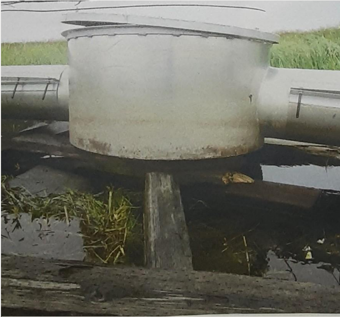
The cold climate water system is sinking due to thawing permafrost.
