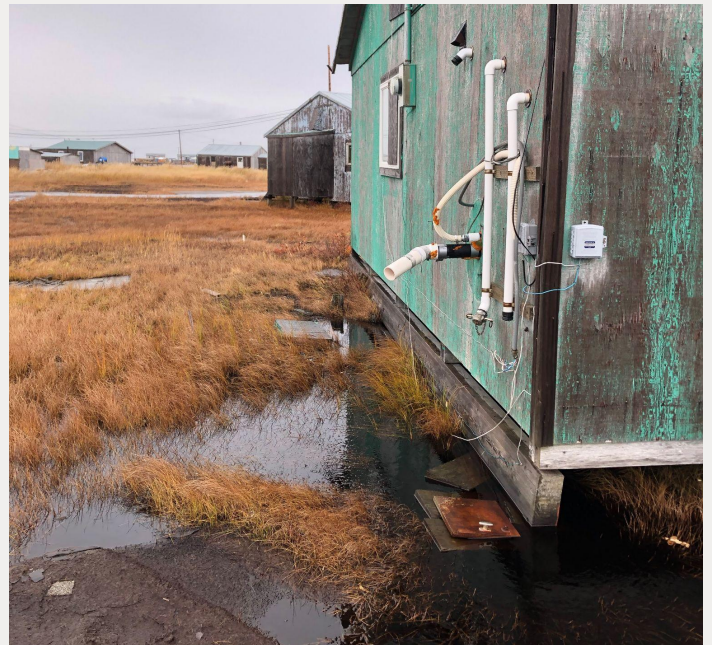
Even in calm weather, water is inundating the foundations of homes in the community due to subsidence from permafrost thaw.
