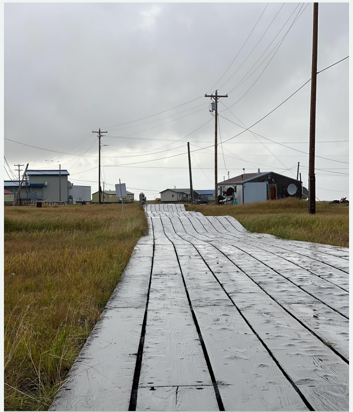
Uneven subsidence of the boardwalk is visible.
